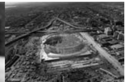
Construction of Superdome
